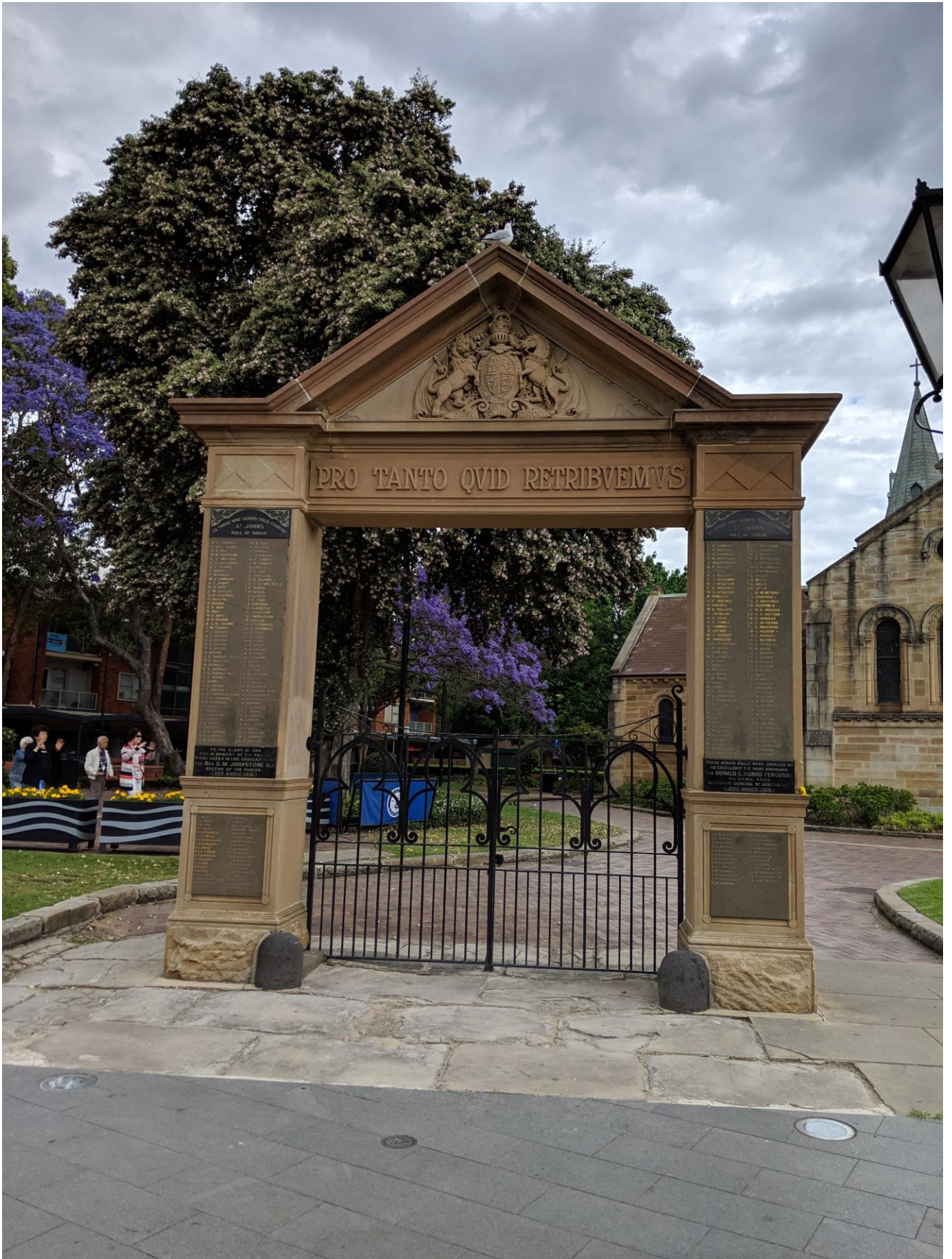
St. John's Anglican Cathedral Memorial Arch Parramatta
